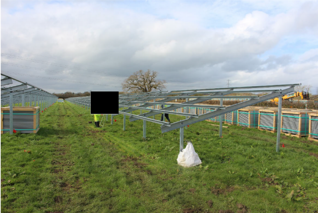
Plate 11d: Installation of Mounting Structures (4 of 4)
