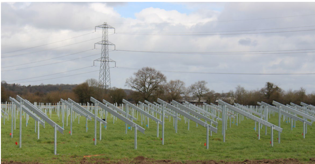
Plate 11c: Installation of Mounting Structures (3 of 4)
