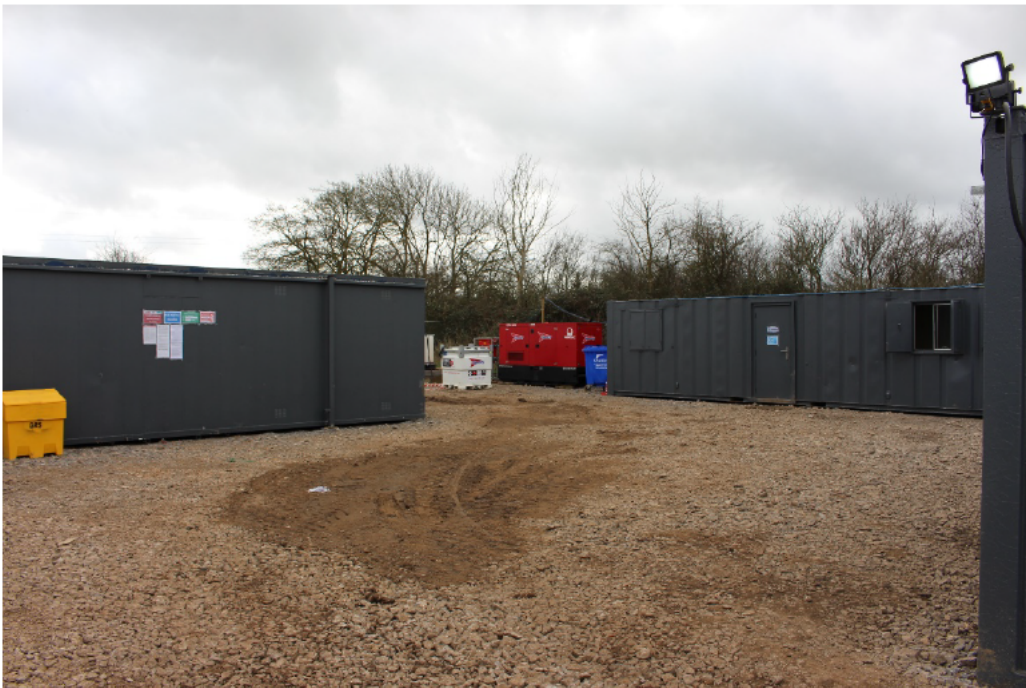
Plate 9: Establishment of the temporary construction compound(s)
