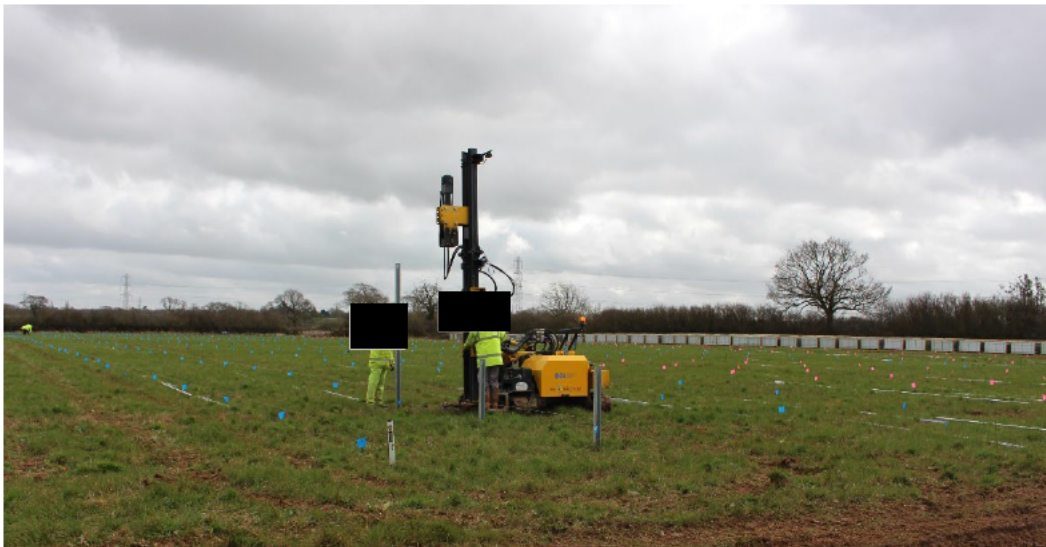
Plate 11a: Marking out location of the infrastructure and installation of Mounting Structures (1 of 4)
