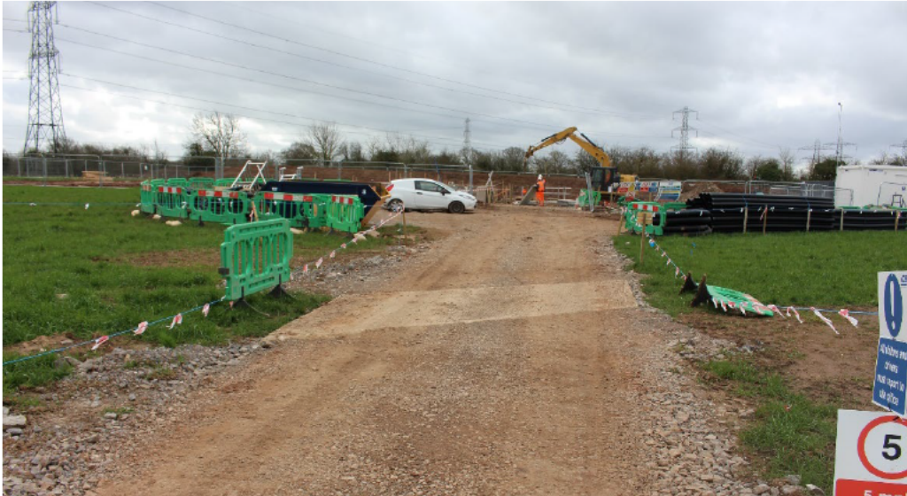
Plate 10: Internal access track and crossing of underground utilities
