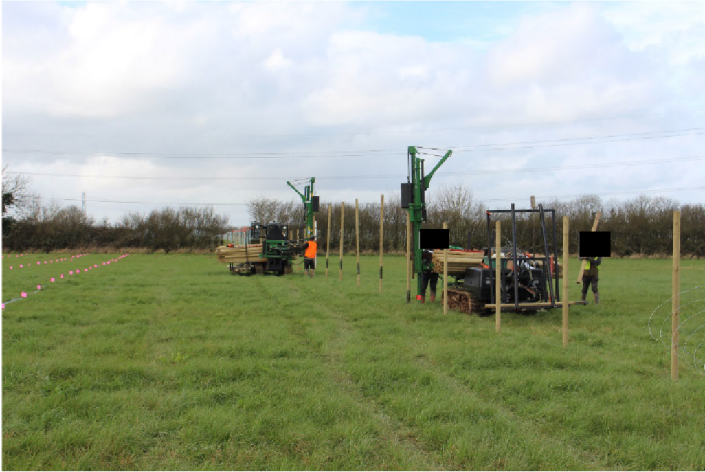
Plate 8: Establishment of Site fencing
