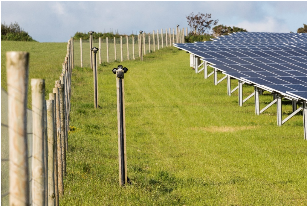
Plate 5: Example of security fencing and monitoring cameras
