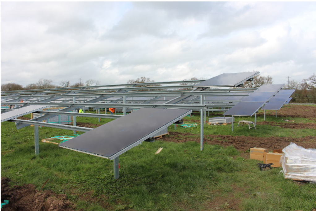
Plate 12: Mounting of PV Modules
